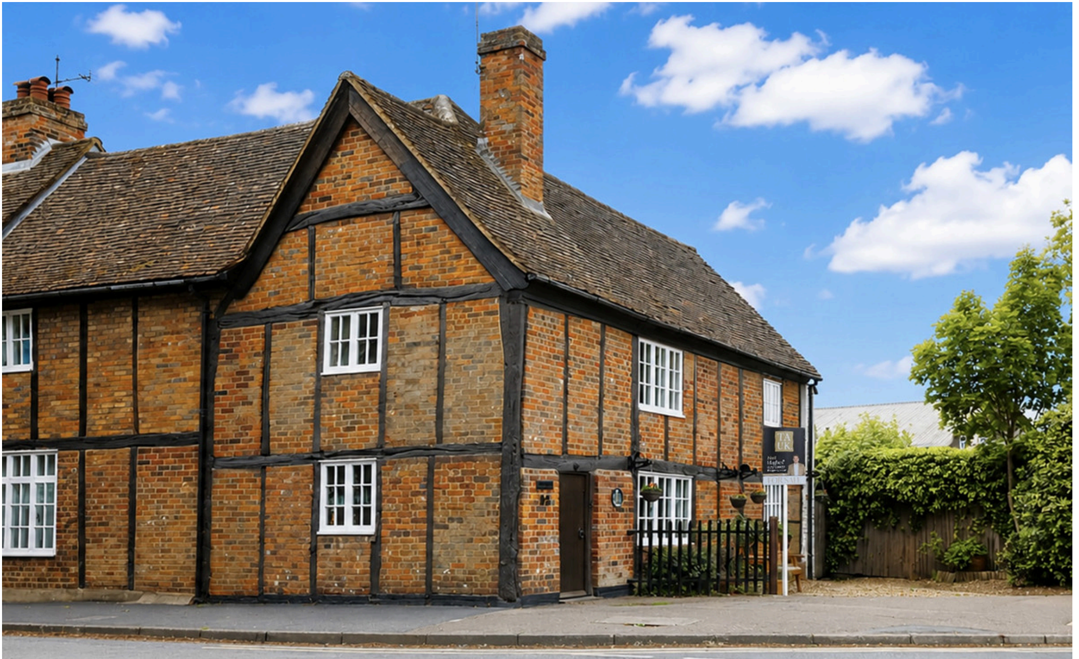
Rose Cottage, Park Street, St. Albans, Hertfordshire, AL2
